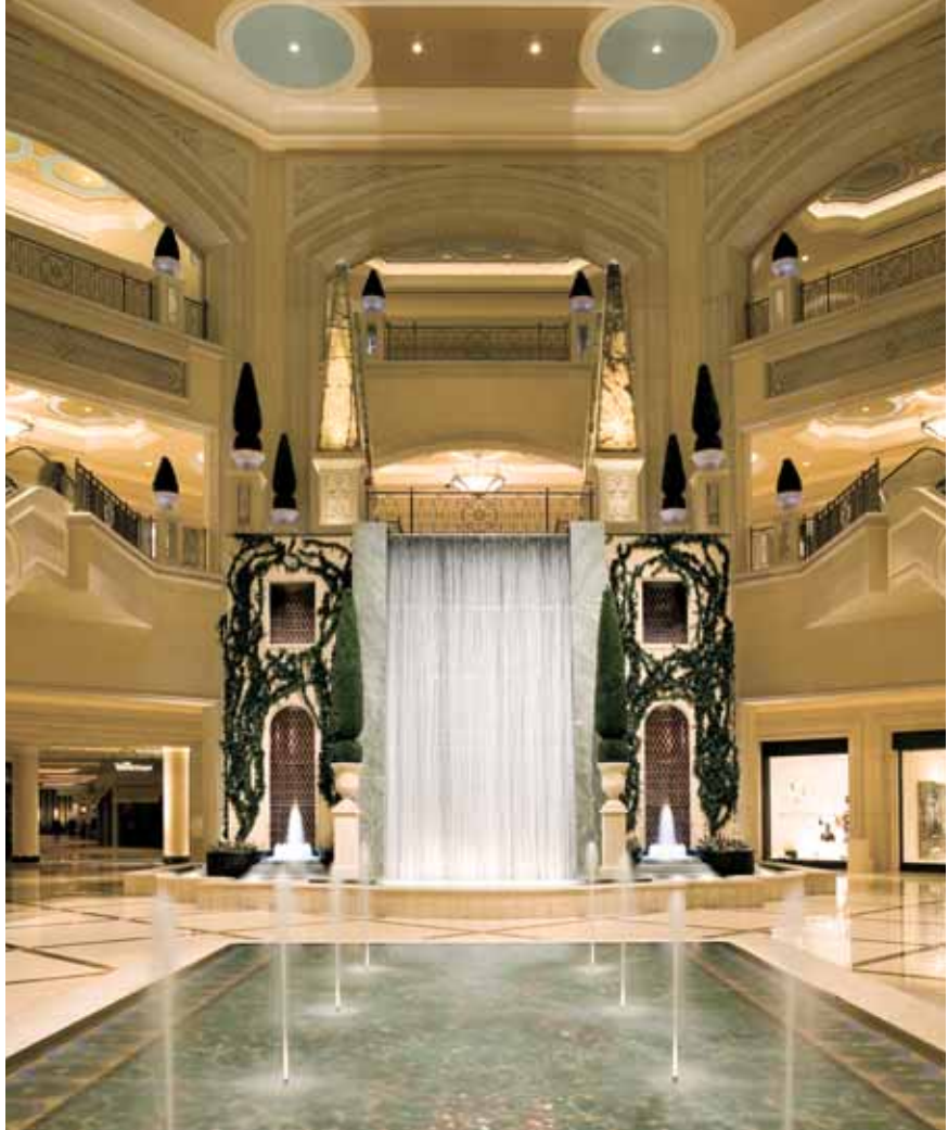
Air quality sensors in densely occupied areas ensure that enough outside air is brought into every conditioned area of The Palazzo. Photo by Blake Marvin/HKS, Inc.
